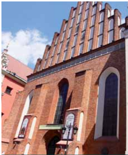
The façade of the cathedral only resembles the Gothic style – there is a concrete structure underneath the brickwork.
